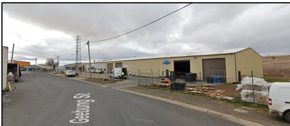
Figure 4: Emergency Services facility adjoining western boundary of subject site
